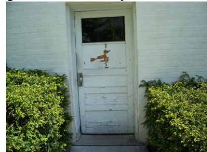
Fig. 21 - Weatherize exterior doors.
