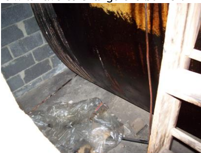
Fig. 7 - The oil tank must be brought up to current NYC DOB Code.
