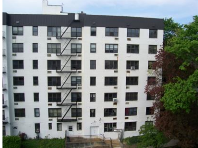
Fig. 10 - Consider replacing windows or sealing them to reduce heat loss.
