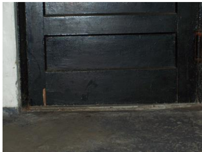
Fig. 16 - Weatherize exterior doors.
