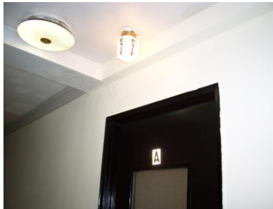
Fig. 32 - Install sensor to avoid having outdoor light on 24/7.
