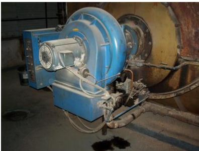
Fig. 4 - Whether the building switches to No. 2 oil or natural gas, it will have to change the burner.
