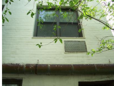
Fig. 11 - Seal through-the-wall A/C sleeves. Insulate unused sleeves.
