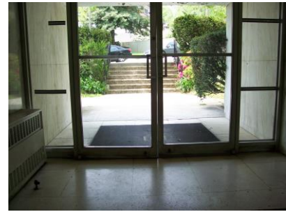
Fig. 15 - Weatherize exterior doors to reduce heat loss.
