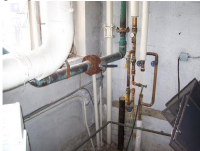
Fig. 29 - Insulate all hot water and steam pipes.
